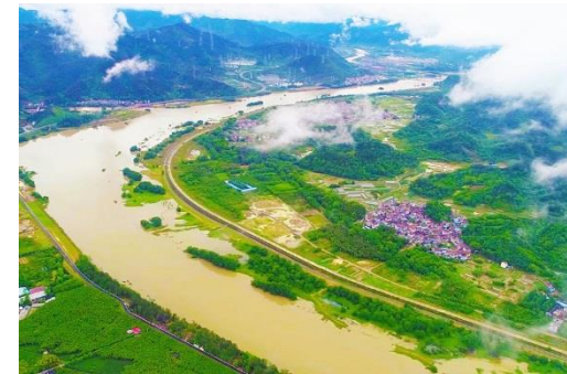
Daxi Environmental Improvement and Upgrading Project in Lishui, Zhejiang
