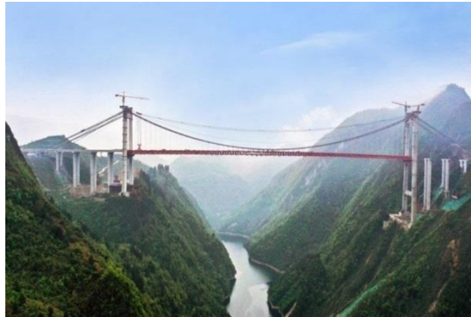
Guiyang - Huangping Expressway Baoshan Super Bridge
