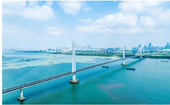
Nanjing Jiangxinzhou Yangtze River Bridge
