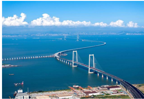
Subsea Tunnel of Shenzhen-Zhongshan Bridge
