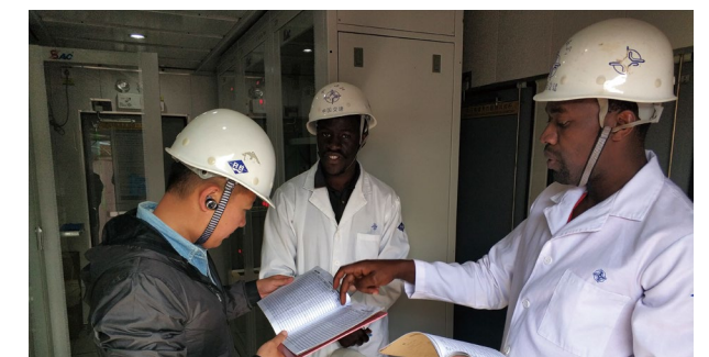
第九项目经理部开展安全检查 Safety Inspection conducted by the Section 9
