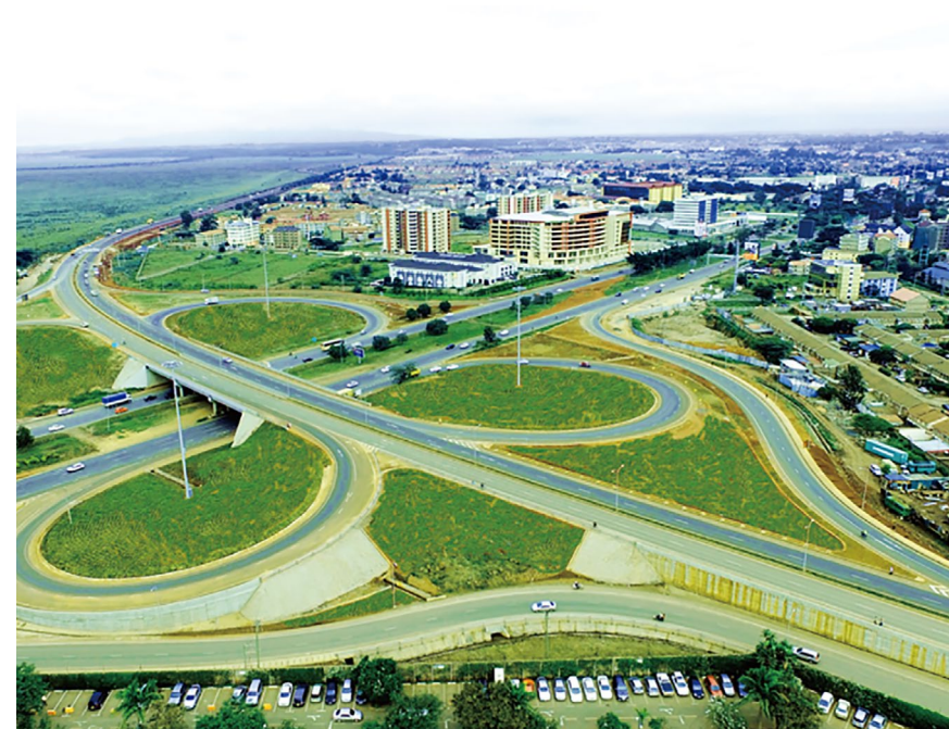
肯尼亚内罗毕南环公路 Kenya Nairobi Southern Bypass
