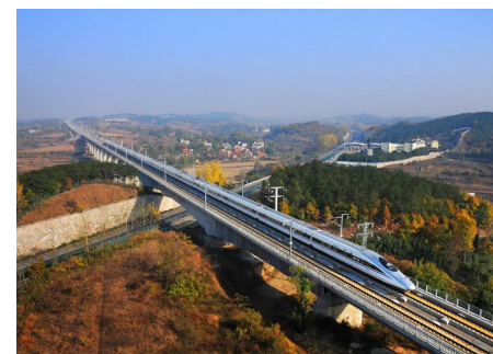
京沪高速铁路 Beijing-Shanghai High-speed Railway
